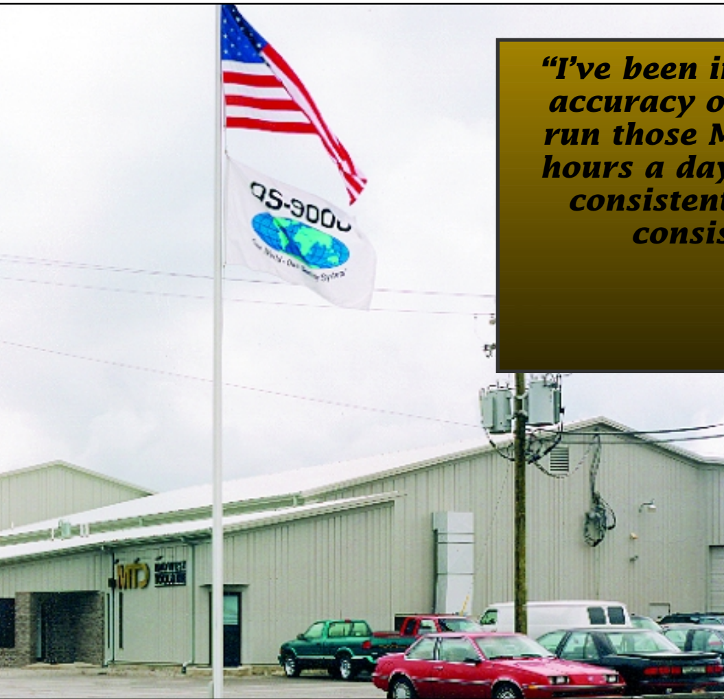
Corporation's manufacturing facility in Fort Wayne, Indiana.
