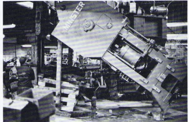
New Minster E2-400 HeviStamper press being installed.
